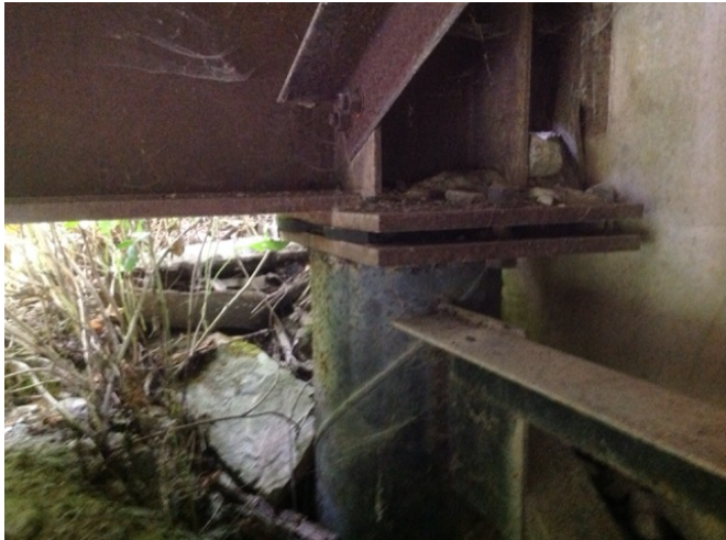
upstream left bearing
