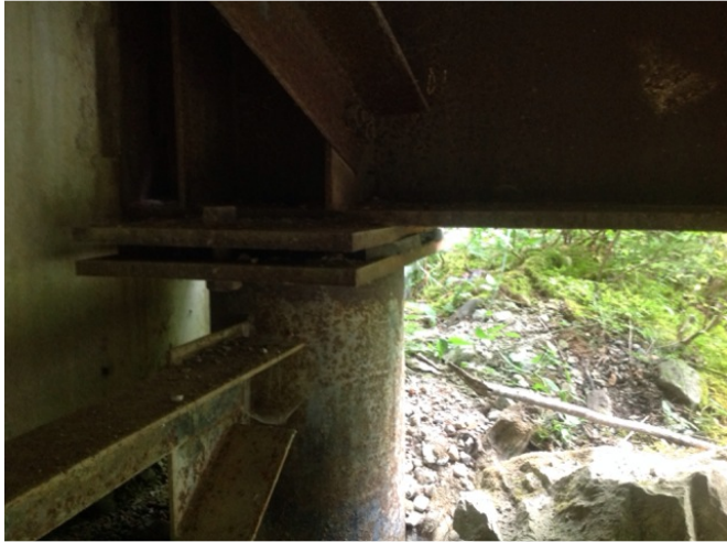
upstream right bearing pads
