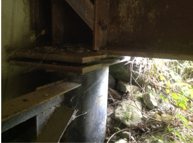
downstream left bearing
