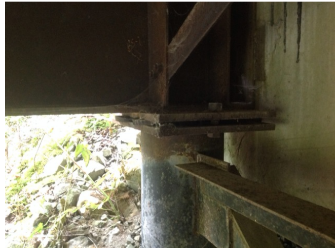
downstream right bearing pads
