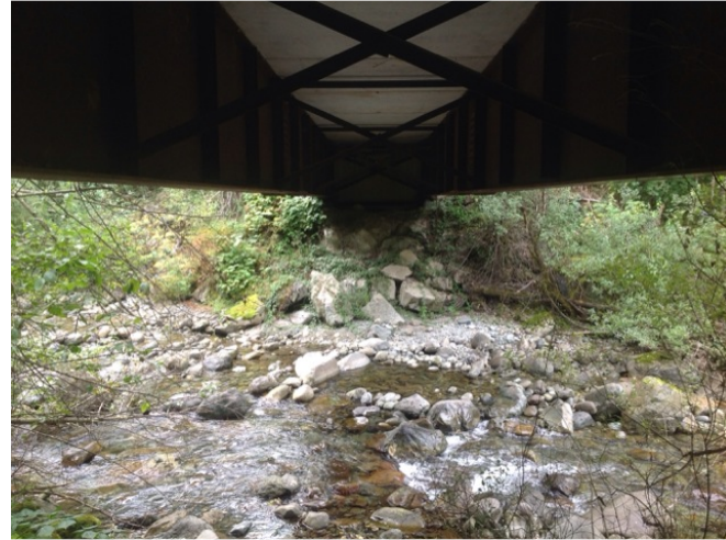
Left Bank Abutment when facing downstream
