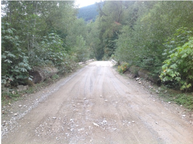
Approach from Left Bank when facing downstream
