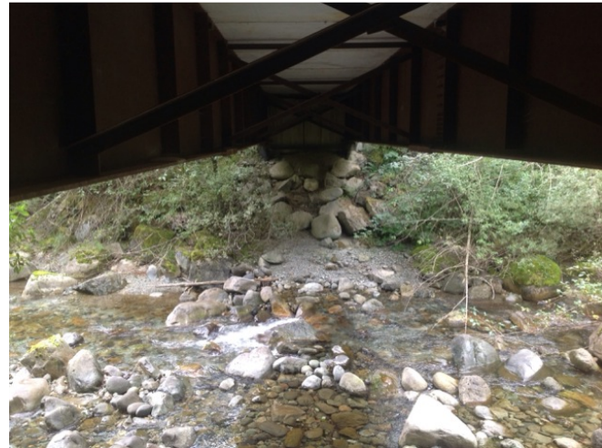
Right Bank Abutment when facing downstream
